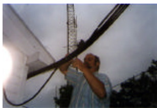
A NERA volunteer rigs the coax on the Fork Mountain 443.250 linked machine.
